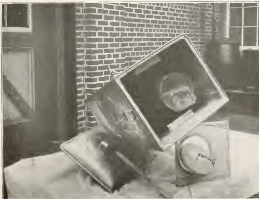
In order to insure that the drinking water is uncontaminated, the water containers are sterilized with live steam. The ice is kept in a separate compartment and does not come in contact with the water.
